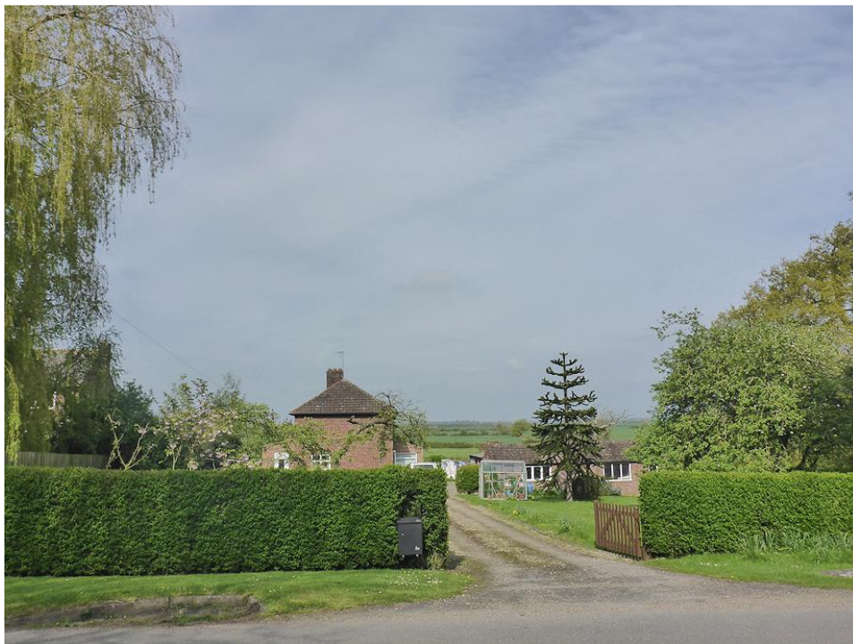
Park Farm Cottage looking west from Fenton Road.
