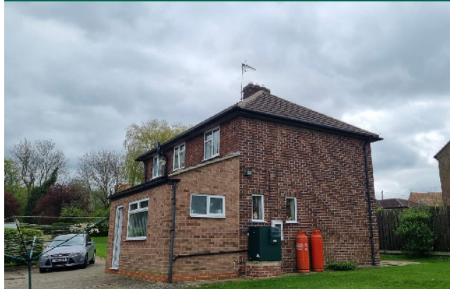
Figure 7 East elevation of Park Cottage
