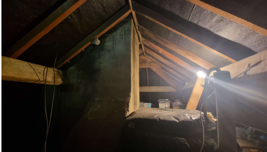
Photo 2: B1 internal roof void showing bitumen underfelt.
