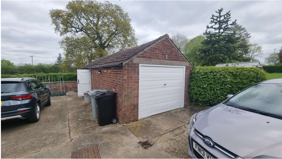
Photo 2: B2 From the Southern Aspect
